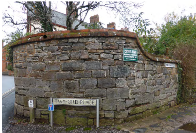
Figure 78: A private garden is enclosed by a rubble stone wall
