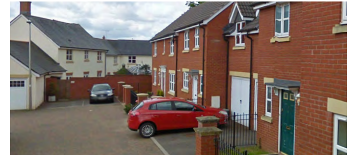
Figure 69: Hayne Court facing south east.
