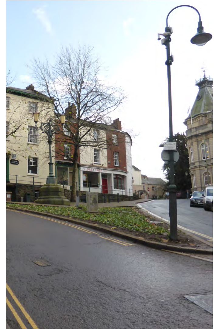
Figure 130: A Traffic island at Junction with St peter street includes street furnitures and listed lamp standard
