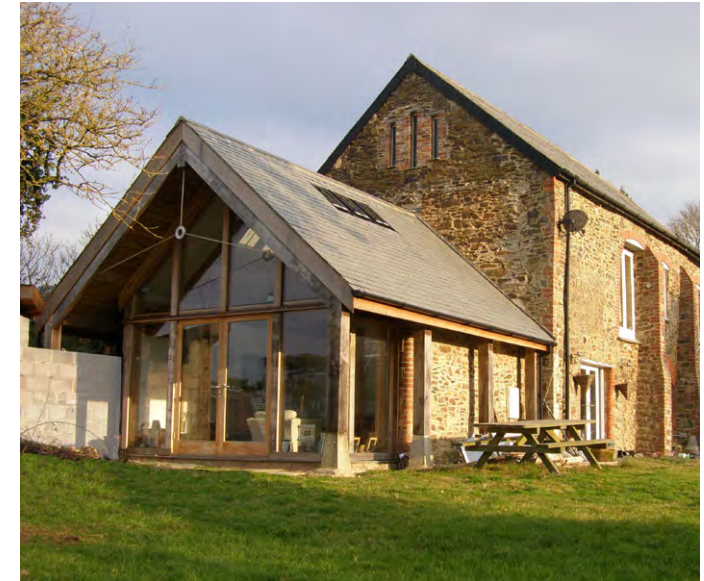
Figure 132: Barn extension at The Granary, Teignbridge ©Living Space Architect
