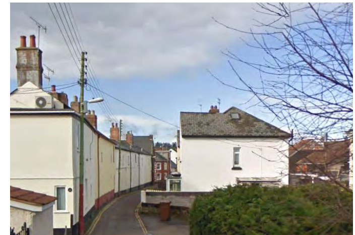
Figure 54: Water Lane facing west.
