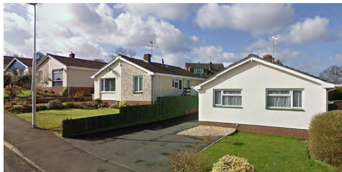
Figure 30: Bungalow housing along Pinnex Moor Road.
