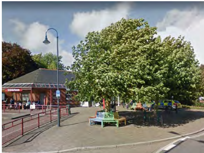
Figure 129: Phoenix Lane - A hard paving open space with trees and street furniture
