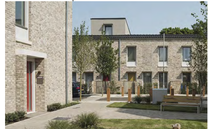
Figure 92: An example showing privacy strip in green corridors, Goldsmith Street, Norwich.
