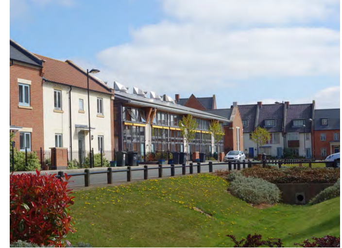
Figure 118: An example of a SuDS corridor - Upton Urban Extension, Northampton
