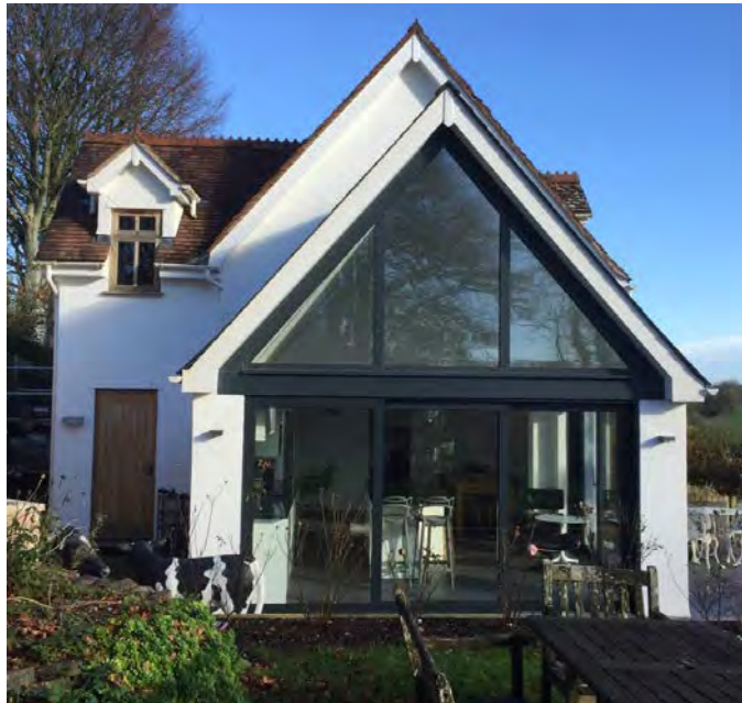
Figure 131: A contemporary extension to a Cottage in Stoodleigh, Devon ©Living Space Architect
