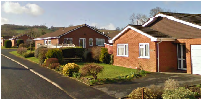
Figure 64: Follett Road facing south.
