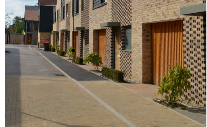
Figure 91: An example showing privacy strip in mews and shared surface streets, Abode, Cambridge.
